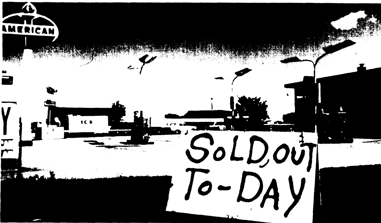
Photo Credit U S Department of Energy
