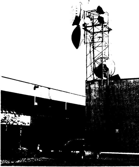
Microwave and satellite dishes at the University of Alaska at Anchorage.
