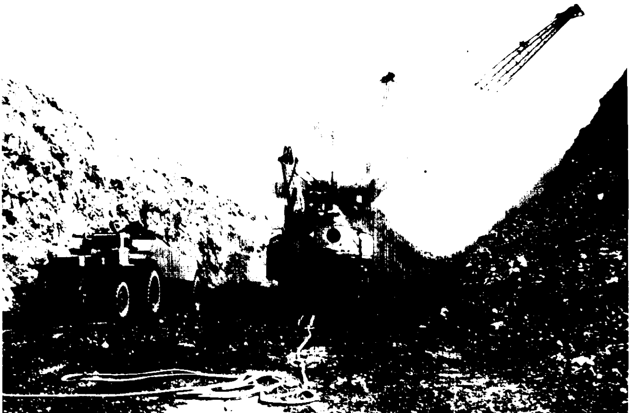
Photo credit: U.S. Department of Energy
