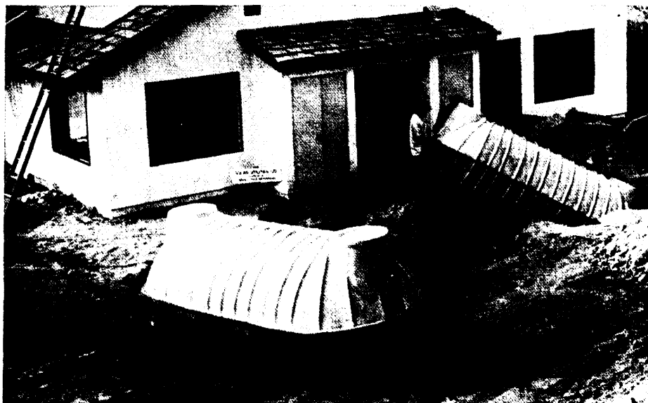
Figure XI-4.— Installation of Fiberglass Underground Tanks
