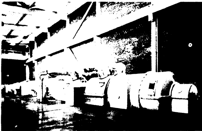
(1) District heating turbine plant delivered by STAL-LAVAL
