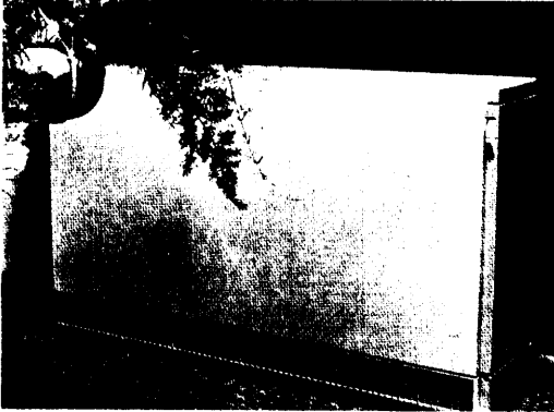
A storage/heating unit installed in a home
