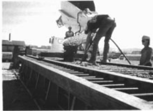
Placing and vibrating concrete
