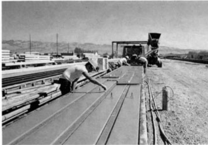
Screeding and finishing surface of pretensioned concrete piles.
